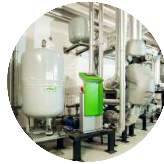
Monitoring of water consumption by modern meters
